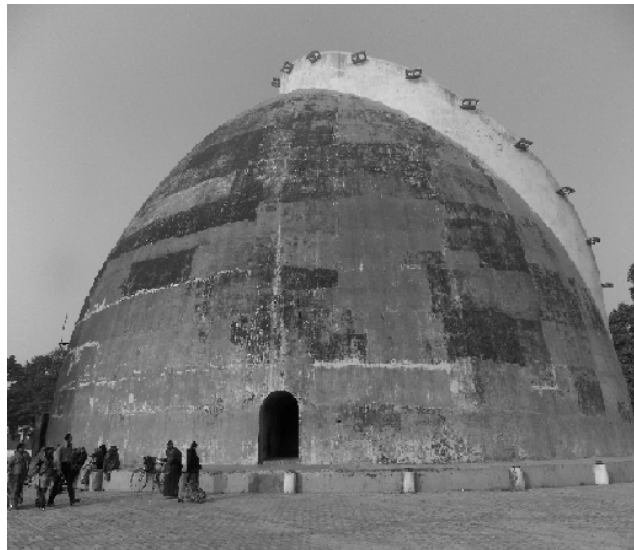
FIG. 1 GOLGHAR COMPLETED IN YEAR 1786 BY THE EAST INDIA COMPANY TO STORE GRAIN [COURTESY UDAY AND SANGEETA VARMA]
