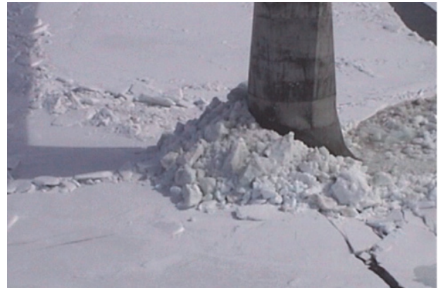
Figure 6: Ice Buildup on Confederation Bridge Piers (Newhook and McGuinn, 2007)
