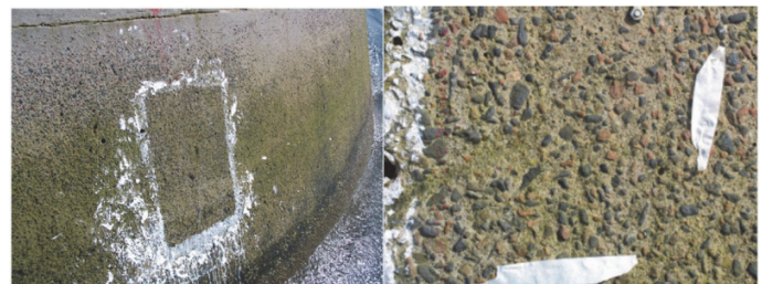
Figure 1: Abrasion of Confederation Bridge Piers (Newhook and McGuinn, 2007)
