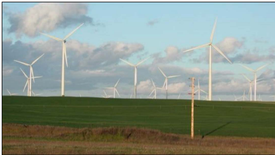
Figure 2.8 – LWT wind farm in California (source: http://en.wikipedia.org/wiki/Wind_farm )
