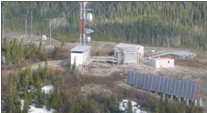
Figure 3.3 – Mulligan, one of Bell-Aliant’s hilltop telecommunication sites
