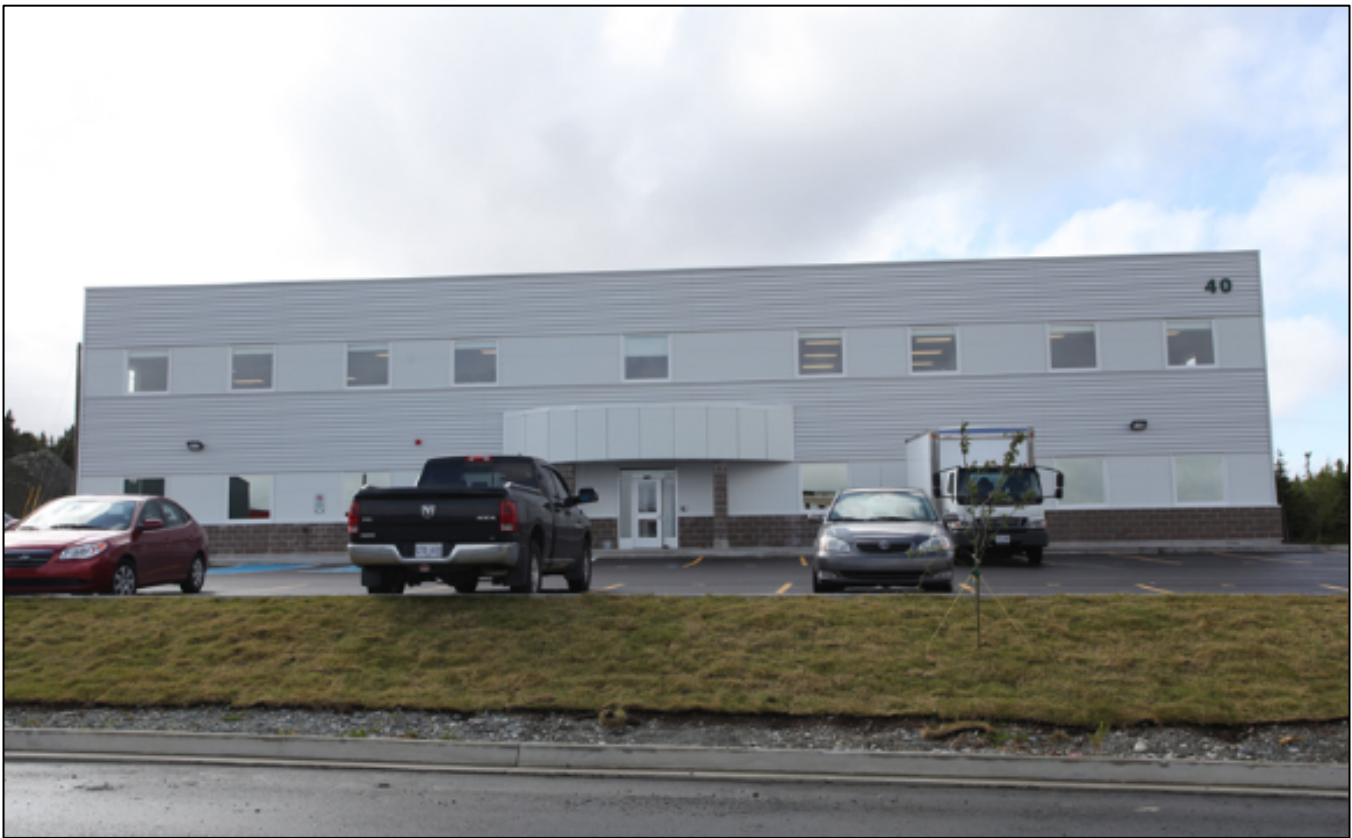
Figure 1.1 – Completed New Office Building Project
