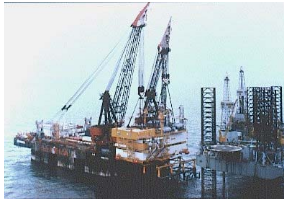
Slide 6 : Installation of 60MN K12-BP topside by floating crane
