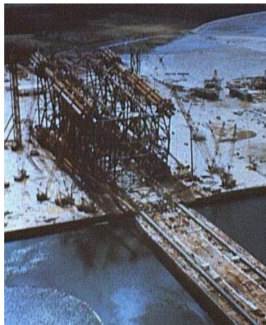
Slide 5 : Jacket being loaded onto barge by skidding
