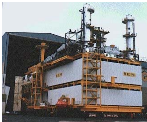
Slide 4 : Integrated topside during load out
