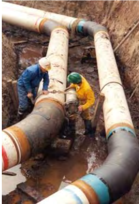
Figure 5. New, large diameter pipelines are expanding
