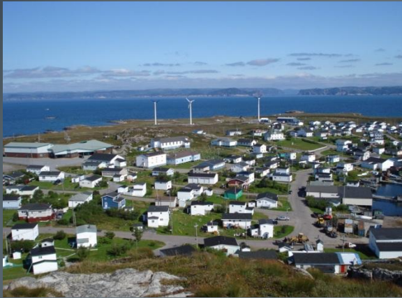
3*100kW Northern power 100 wind turbines in Ramea
