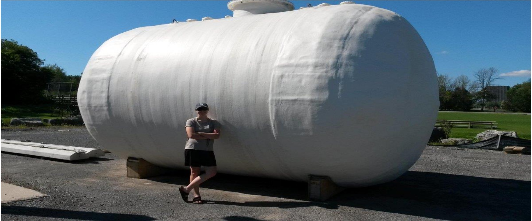
Fig. 01: 35 m 3 below grade STST at Carleton University, Ottawa [3]
