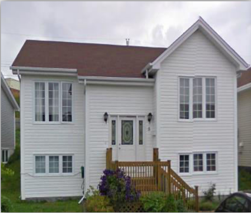
Two storey building with a semi finished basement and fully finished first floor (house-1).
