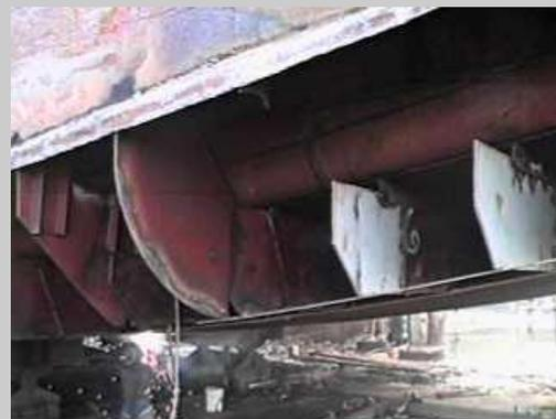
**Frames** in the **void** wing tank of a river barge. In this photo, the knuckle plate has been cut away so that bent frames can be renewed. The **double bottom** is exposed. New knuckle plate will be installed once the frames are renewed.
