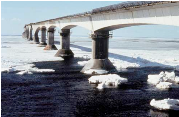
Figure 10.10 Confederation Bridge showing icebreaking cones at the waterline
