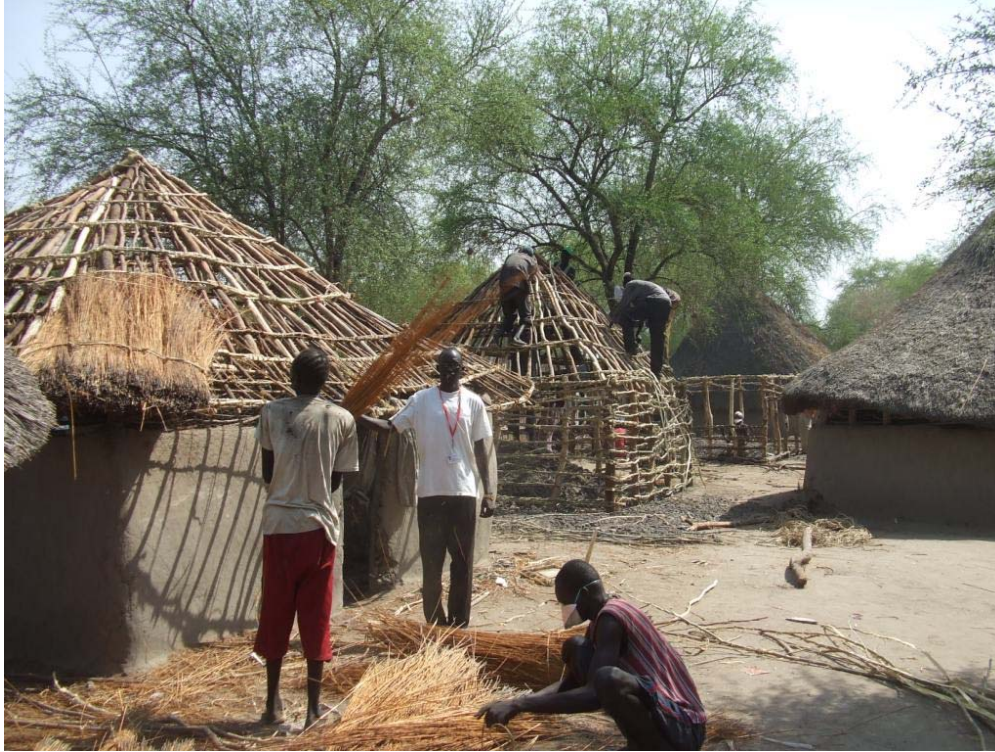
FIGURE 10 TOKUL (TRADITIONAL HUTS) UNDER CONSTRUCTION IN LANKIEN – SIMILAR TO THOSE PROPOSED
