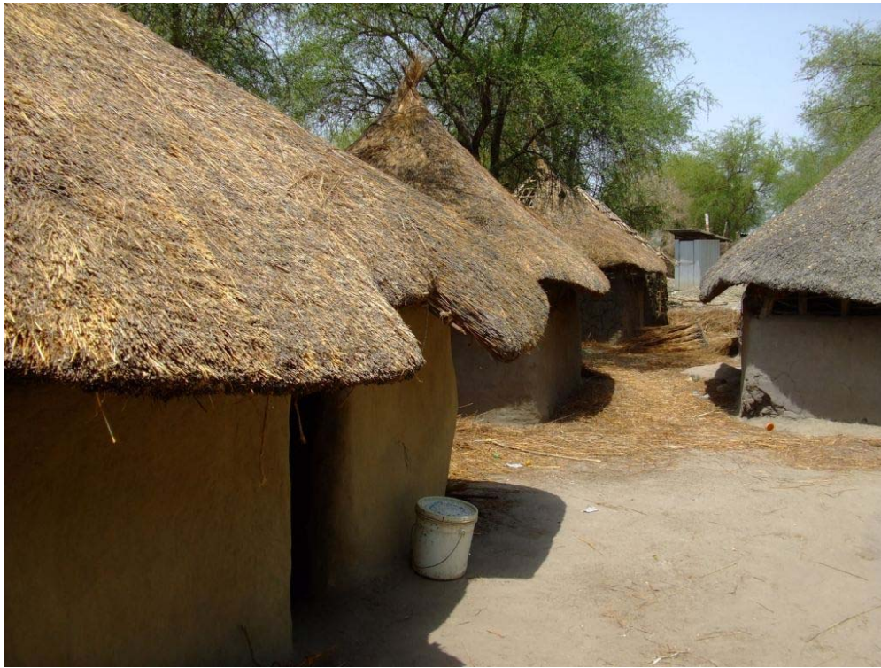
FIGURE 11 SAME HUTS NOW COMPLETE (COURTESY OF MSF LANKIEN)
