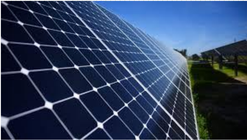
PV Array, Efficiency: 14~18%
