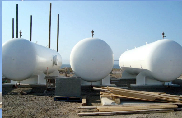
Figure: Three Hydrogen Tanks of 1000 Nm 3 combined Capacity .
