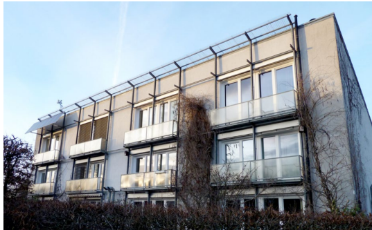
1. The world's first multi-family Passive House, Darmstadt-Kranichstein, Germany 1990
