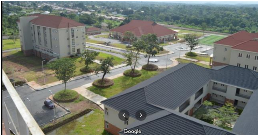
Fig. 1: Overview of part of the University campus.
