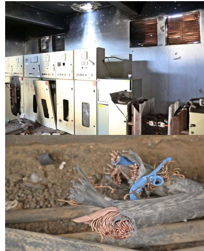
the damage in electricity grid
